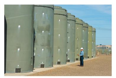
Nuclear fuel is typically used in the reactor for 3-6 years and then must be removed. The rods are highly radioactive and must be stored under water for cooling and radiation shielding. After years in the overcrowded pools, the spent fuel assemblies are moved into dry storage casks which will deteriorate over time.
